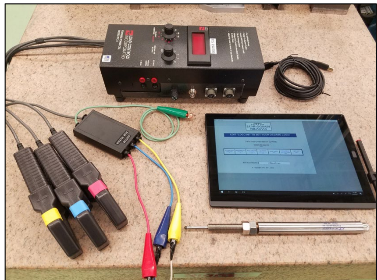
Figure 3: Field Instrumentation System used to measure three-phase spindle grinding power
